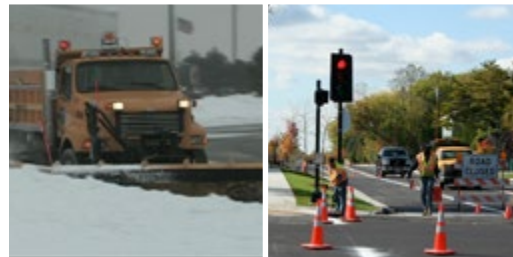
20% will be invested in public works services, such as snow plowing, road maintenance and similar work
